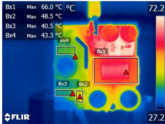
Figure 31 – Top Thermal Image, T_{AMB} = 25.6 °C. Bx1: Transformer, T_1 = 66.0 °C. Bx2: Thermistor, RT1 = 48.5 °C. Bx3: CMC 1, L1 = 40.5 °C. Bx4: CMC 2, L2 = 43.3 °C.
